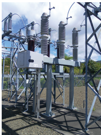
Figure 17.12: Live tank SF 6 outdoor 33kV circuit breaker
