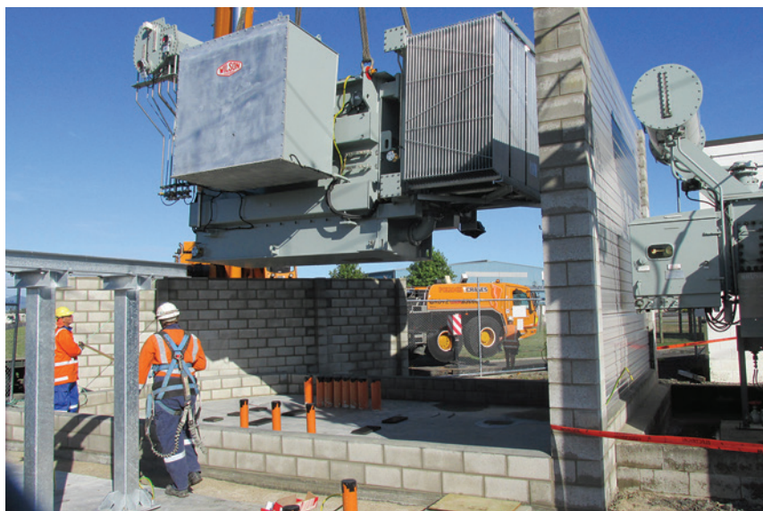
Figure 17.1: Power transformer installation at Waharoa
