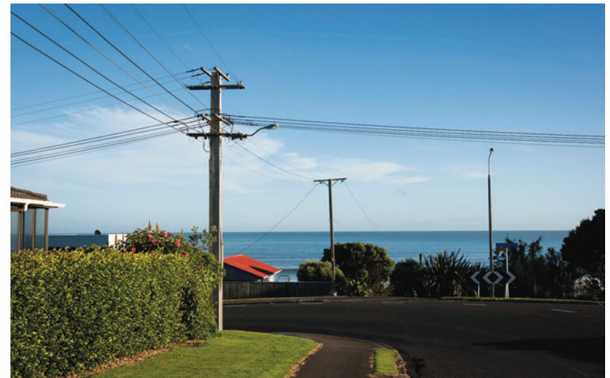
Figure 15.13: LV overhead circuit
