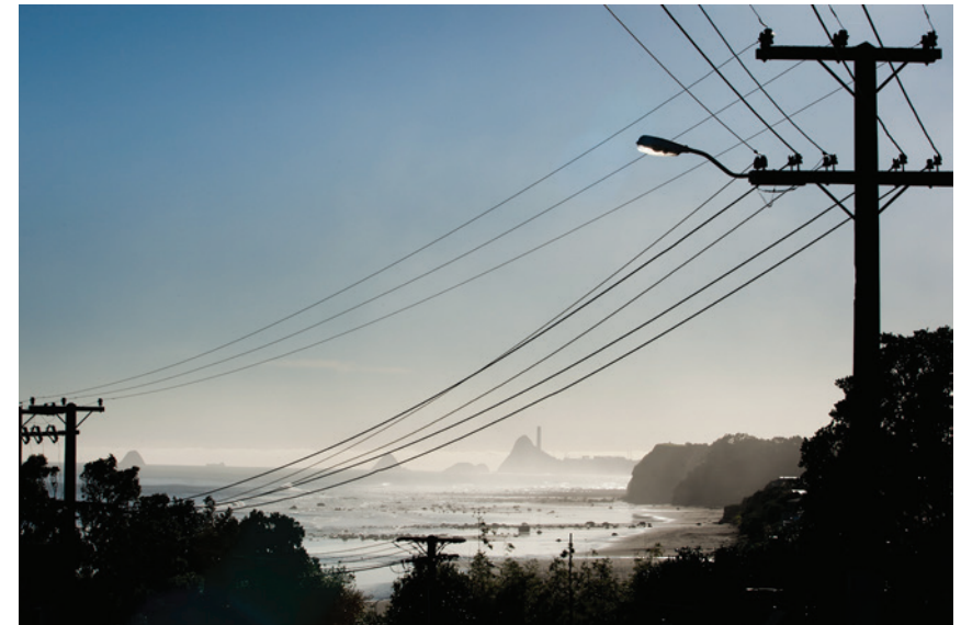
Figure 15.6: Distribution overhead line with LV underbuilt
