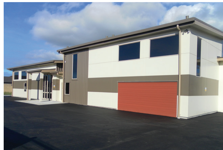
Figure 17.15: Urban zone substation building
