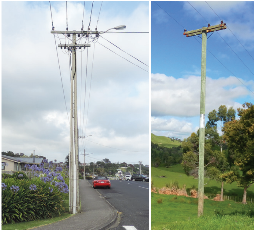
Figure 14.1: A modern pre-stressed concrete pole and a rural softwood pole
