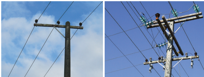
Figure 14.8: Different crossarm configurations
