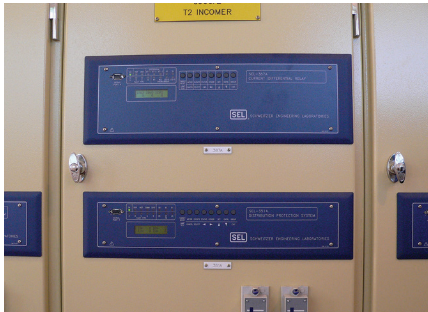
Figure 20.4: Modern numerical relays
