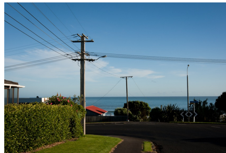
Figure 16.14: LV overhead circuit
