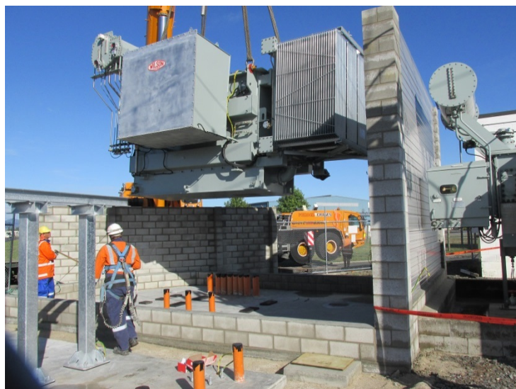
Figure 18.1: Power transformer installation at Waharoa
