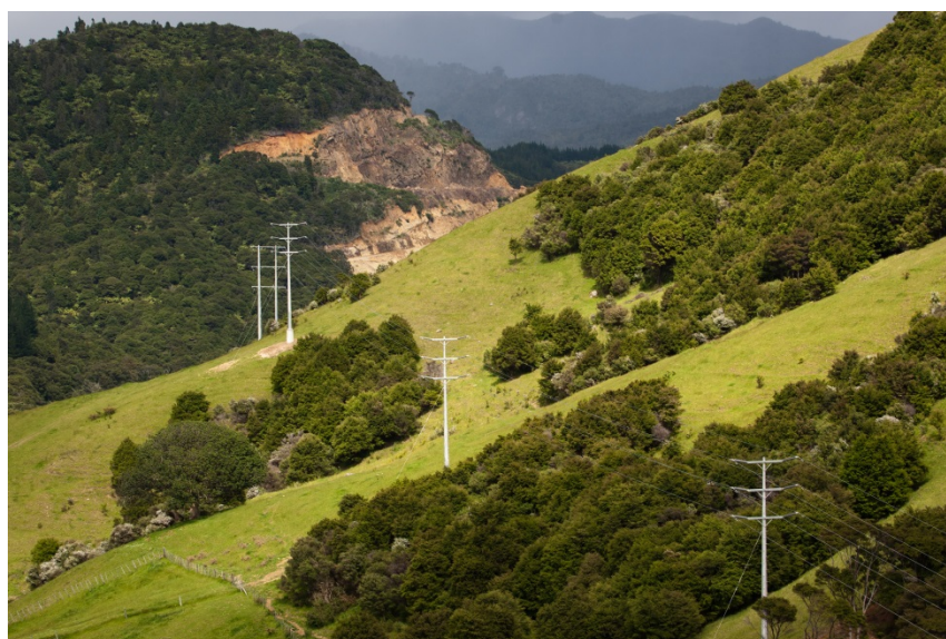
Figure 16.1: 66kV subtransmission overhead line in the Coromandel
