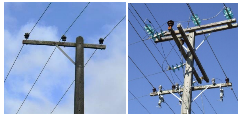
Figure 15.8: Different crossarm configurations
