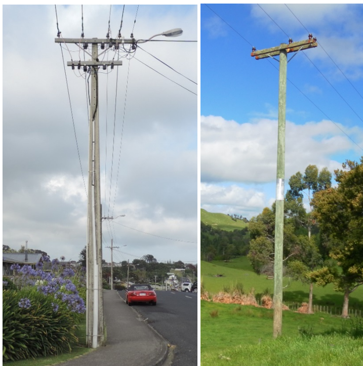
Figure 15.1: A modern pre-stressed concrete pole and a rural softwood pole
