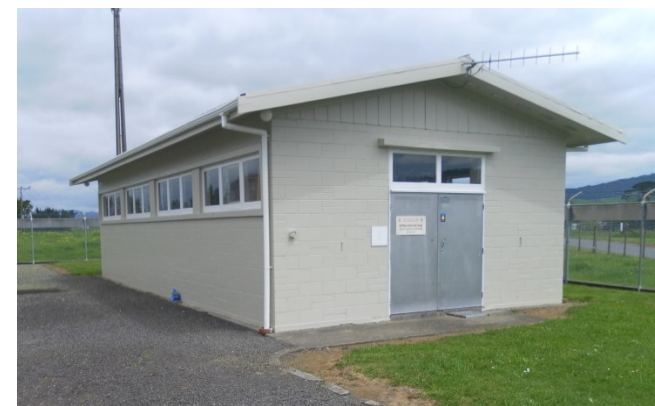
Figure 18.14: Masonry constructed building
