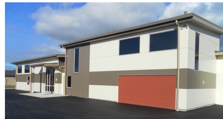
Figure 18.15: Urban zone substation building
