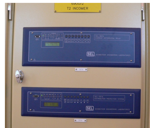
Figure 21.4: Modern numerical relays
