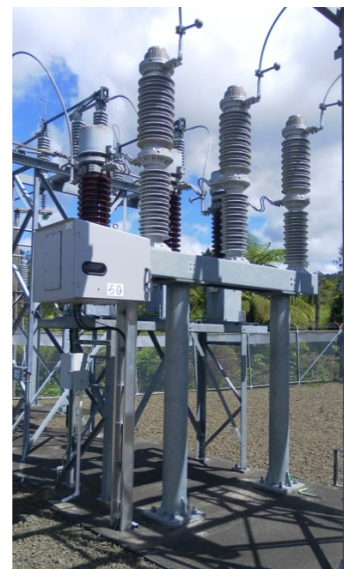
Figure 18.12: Live tank SF6 outdoor 33kV circuit breaker
