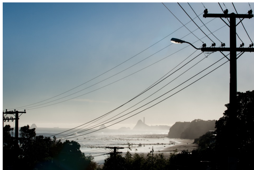
Figure 16.6: Distribution overhead line with LV underbuilt
