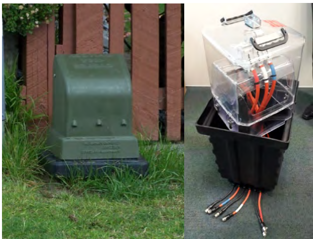
Figure 6.11: Example of organic adaptation. Standard LV pillars (left) are vulnerable to coastal inundation as they are not waterproof. A newer submersible design (shown right).
