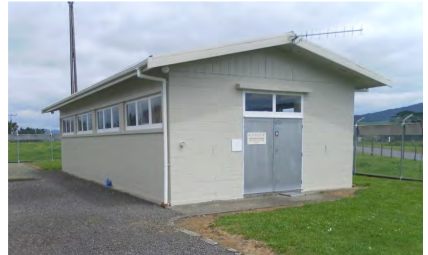
Figure 21.12: Masonry constructed building
