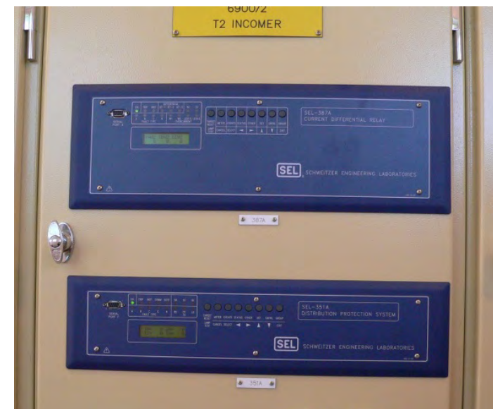
Figure 24.4: Modern numerical relays
