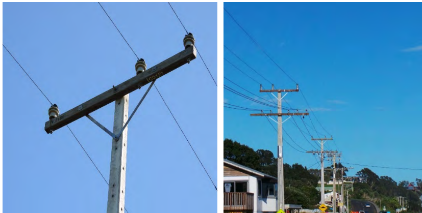
Figure 18.6: Different crossarm configurations
