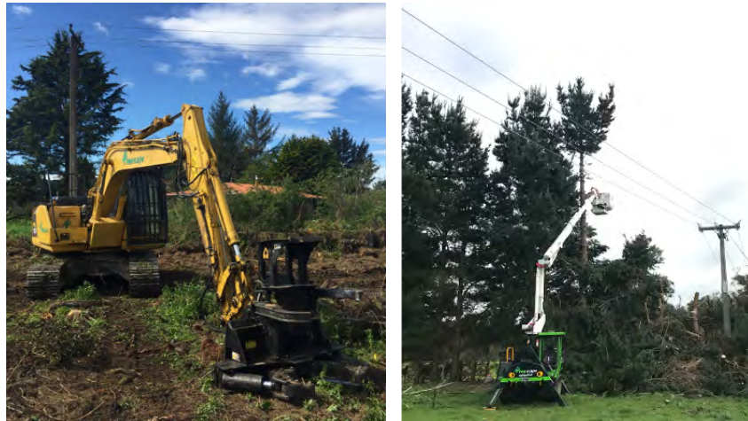
Tree shears provide controlled felling near power lines.
