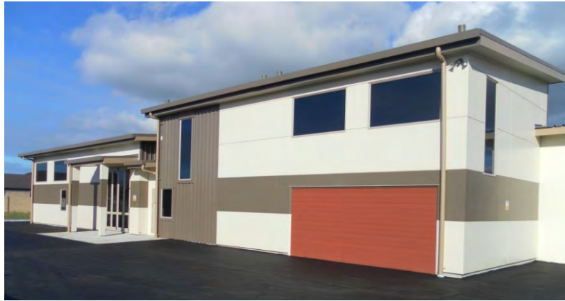
Figure 21.13: Urban zone substation building
