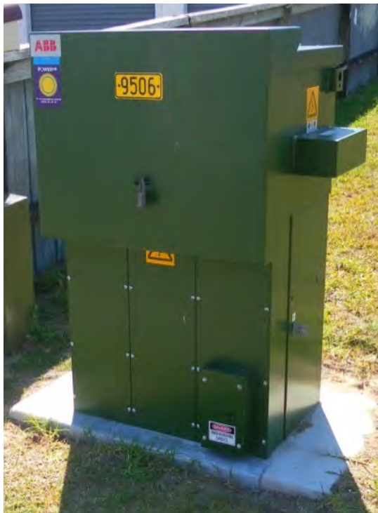
Figure 23.1: Ground-mounted switchgear
