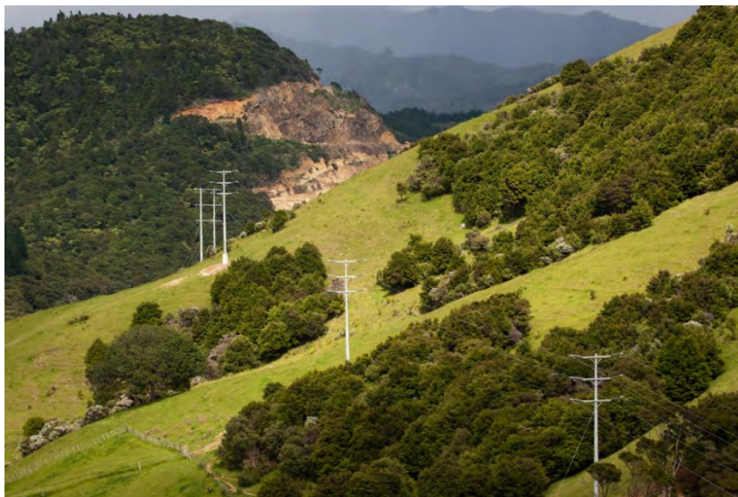
Figure 19.1: 66kV subtransmission overhead line in the Coromandel
