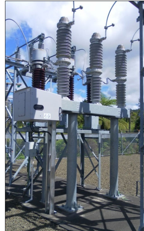
Figure 17.112: Live tank SF 6 outdoor 33kV circuit breaker
