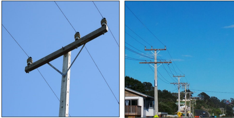
Figure 14.5: Single-circuit and multi-circuit structures
