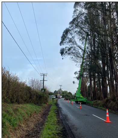
Tree felling near power lines.
