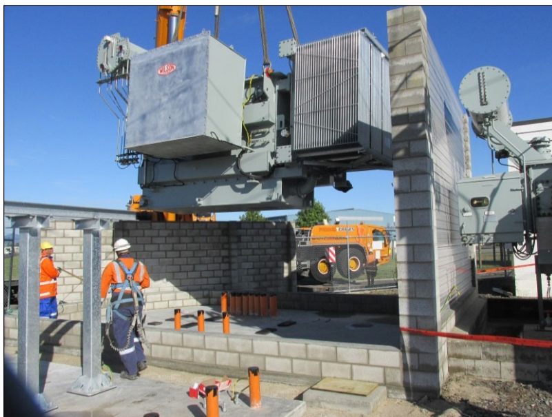
Figure 17.1: Power transformer installation at Waharoa
