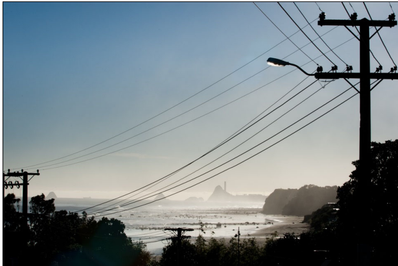
Figure 155.4: Distribution overhead line with LV underbuilt
