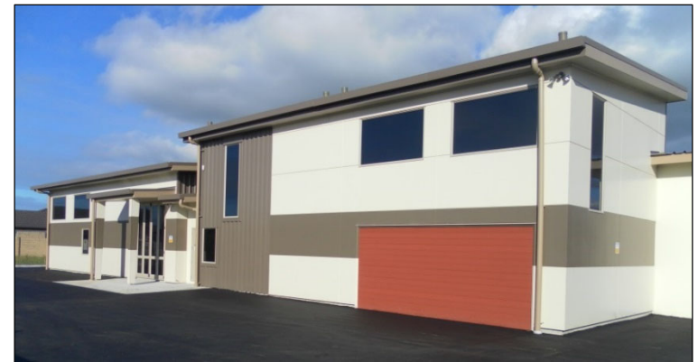
Figure 17.124: Urban zone substation building
