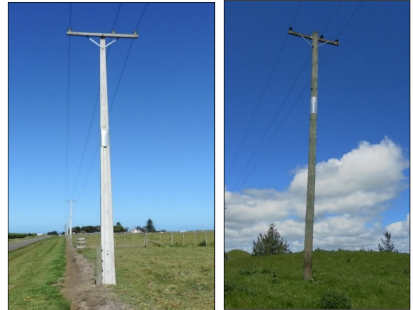
Figure 144.1: A modern pre-stressed concrete pole and a rural softwood pole
